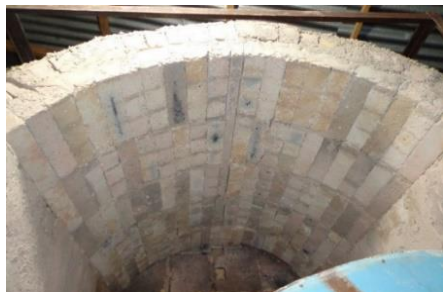
Figure 12. Completed Arch Form
