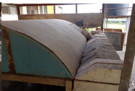
Figure 11. Arranged Skewback on Mould
