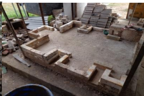
Figure 5. Starting the Kiln Walls
